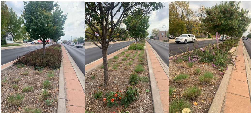
Figure 2 - Site Visit Photographs of Robert Street South, West Saint Paul, MN (Photos by S. Rath)
